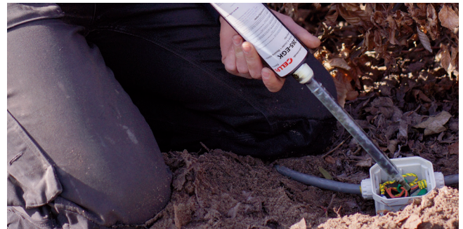
Quick and easy filling with the AMX Resin injection system
